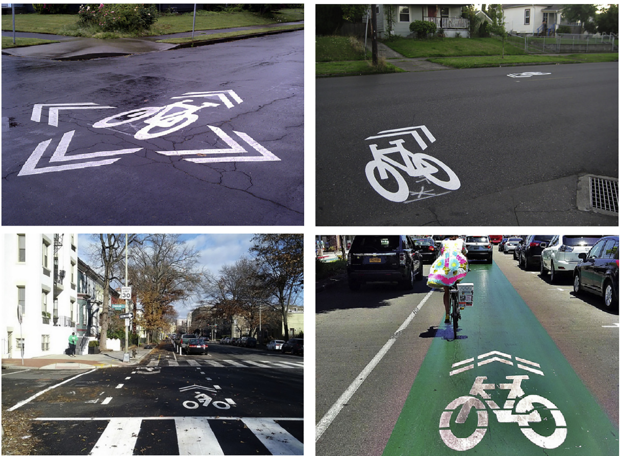
Fig. 3. Examples of alternative forms of sharrows (clockwise from top-left): Portland's Sharrow Flower, a diagonal wayfinding sharrow, Long Beach's Green Sharrow, and an intersection sharrow. Photo Credit: Michael Anderson, NACTO, San Francisco Bicycle Coalition, and Eric Fischer
