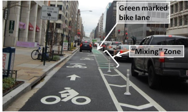
Turning Zone with Post Restricted Entry and Through Bike Lane (TBL)
