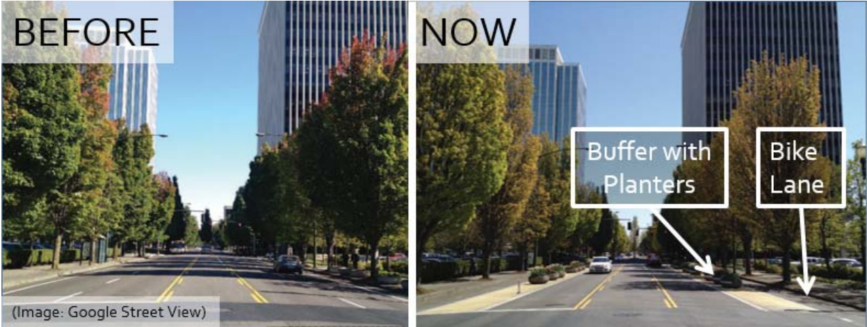
Figure 3-26. NE Multnomah St., Portland, OR, Before and After Installation of Protected Bike Lane
